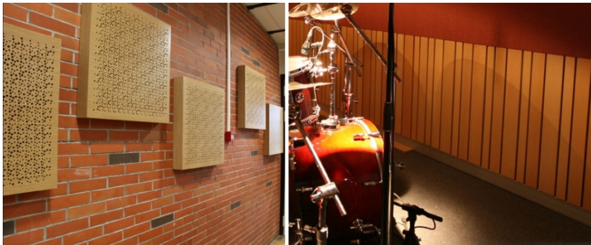
Figure 4.6. Perforated Helmholtz panel ( Acoustissimo , left) and laminar resonator ( Madeinacoustic , right)
