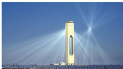
Figure 3.28. Optical losses due to atmospheric attenuation
