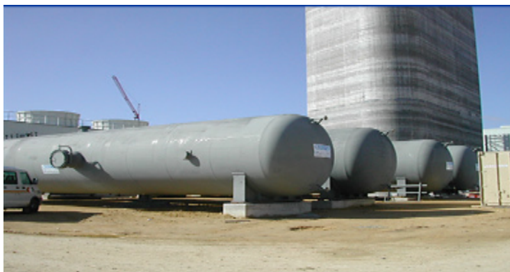
Figure 8.13. Four steam accumulators of the PS10 power plant (Abengoa Solar)
