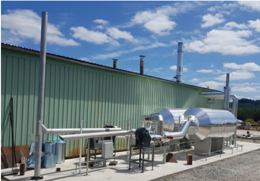
Figure 8.6. Eco-Stock thermocline storage used to store 2 MWh heat on an industrial site (Eco-Tech Ceram)
