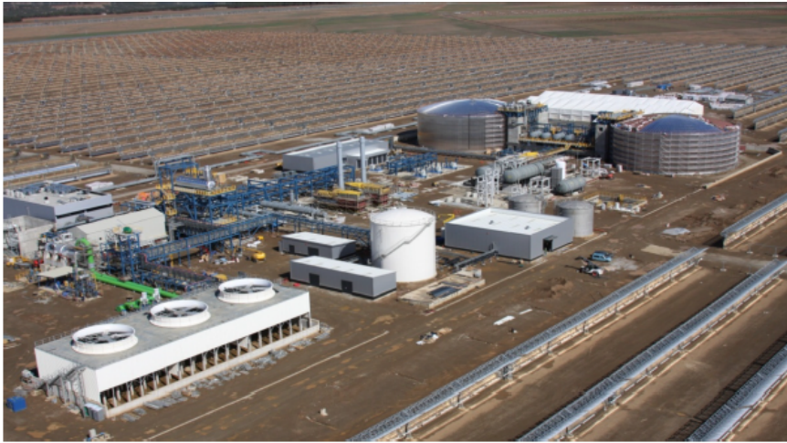
Figure 8.2. Andasol power plant; the storage tanks are visible in the upper right
