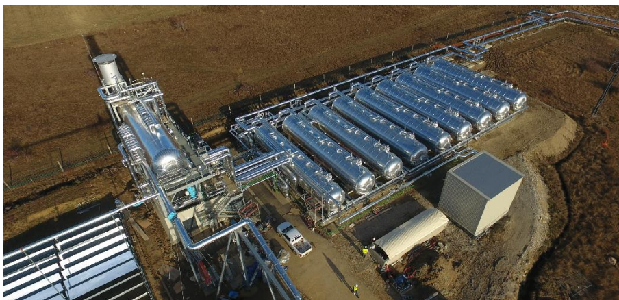
Figure 8.14. Image of the storage tanks of eLLO power plant (SUNCNIM)
