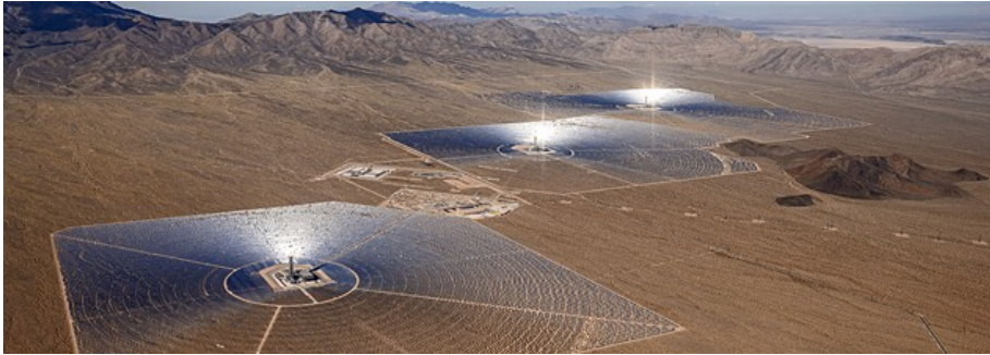
Figure 1.22. Ivanpah solar power plant, three 130 MW e towers (source: BrightSource Energy)
