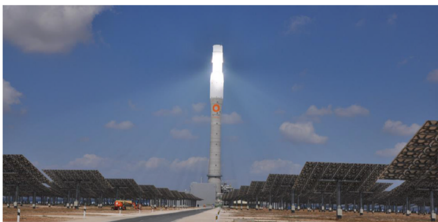
Figure 4.7. Gemasolar, tower power plant with molten salt near Seville, Spain (Ho 2017)
