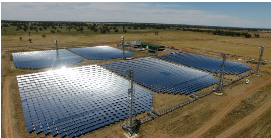
Figure 1.40. Jemalong CSP Pilot Plant, pilot solar power plant using sodium as heat transfer fluid (Vast Solar 2020)
