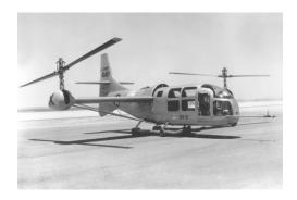
Figure 2. Bell XV-3 Helicopter with two-blade rotor
